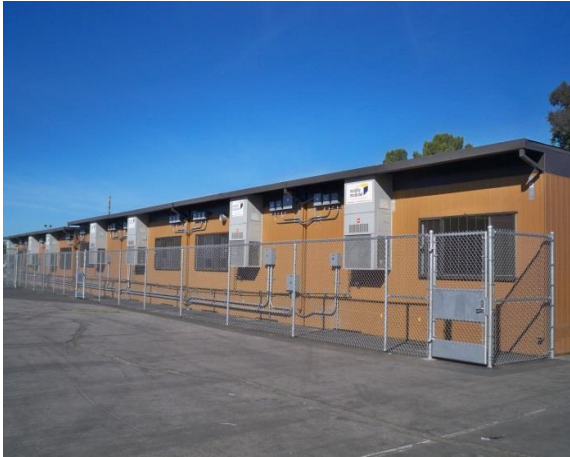
Back of Classroom
