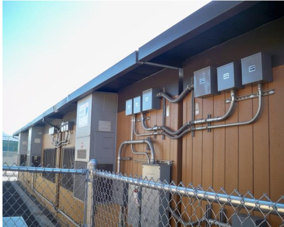
Back of Classroom
