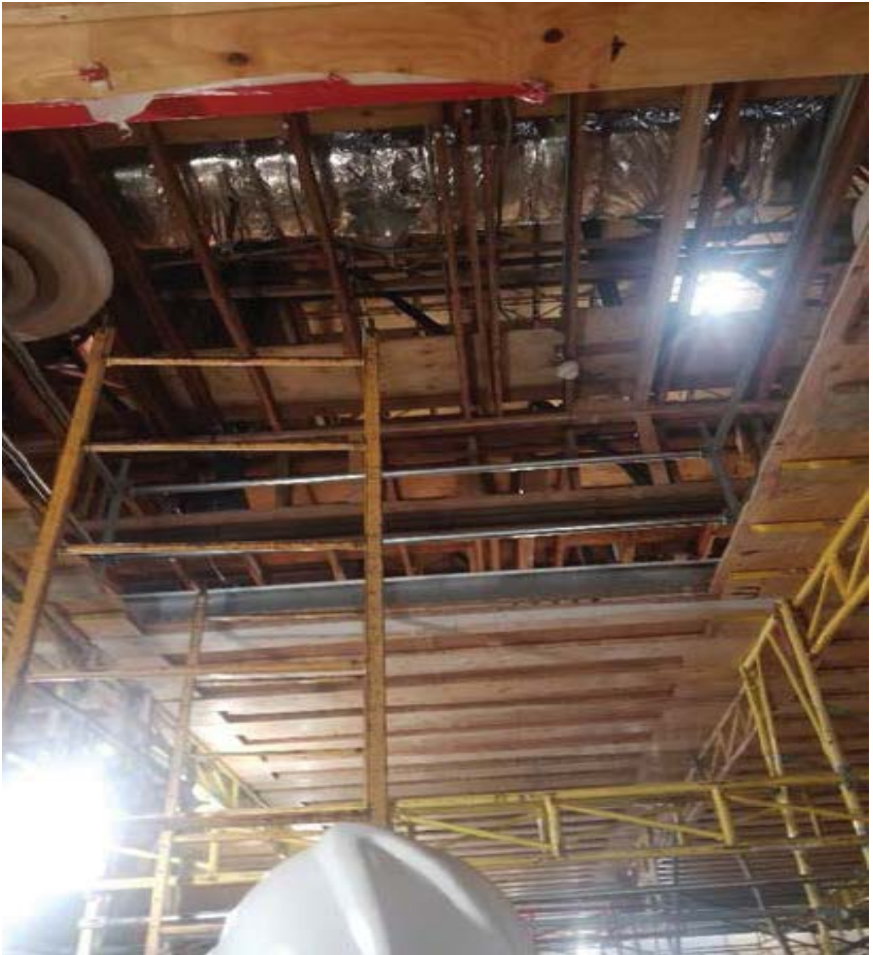
Auditorium Interior Ceiling Renovation in Progress
