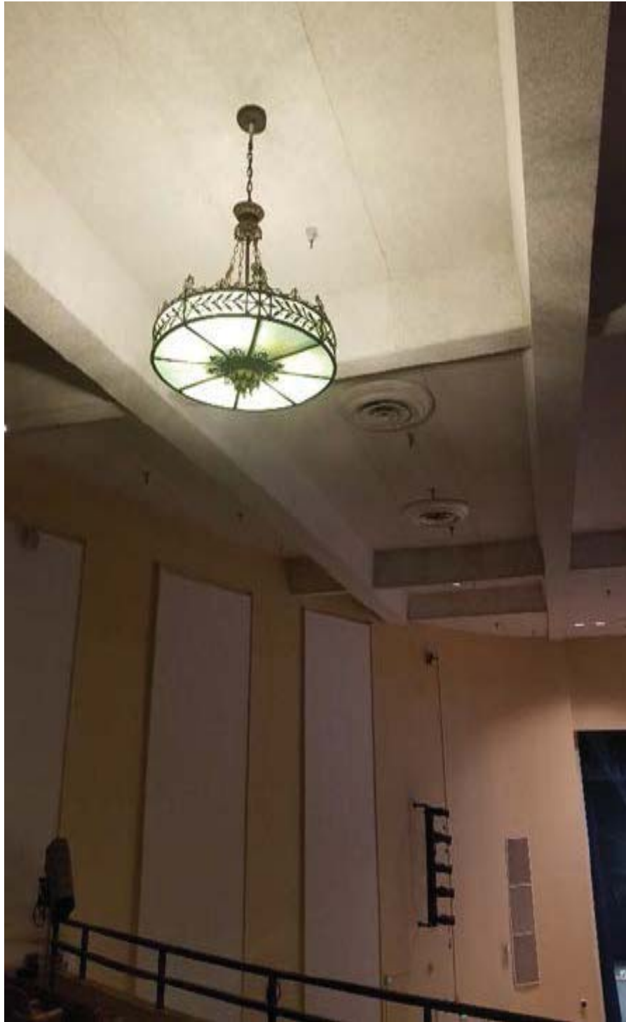
Renovation of the Interior of the Auditorium Ceiling
