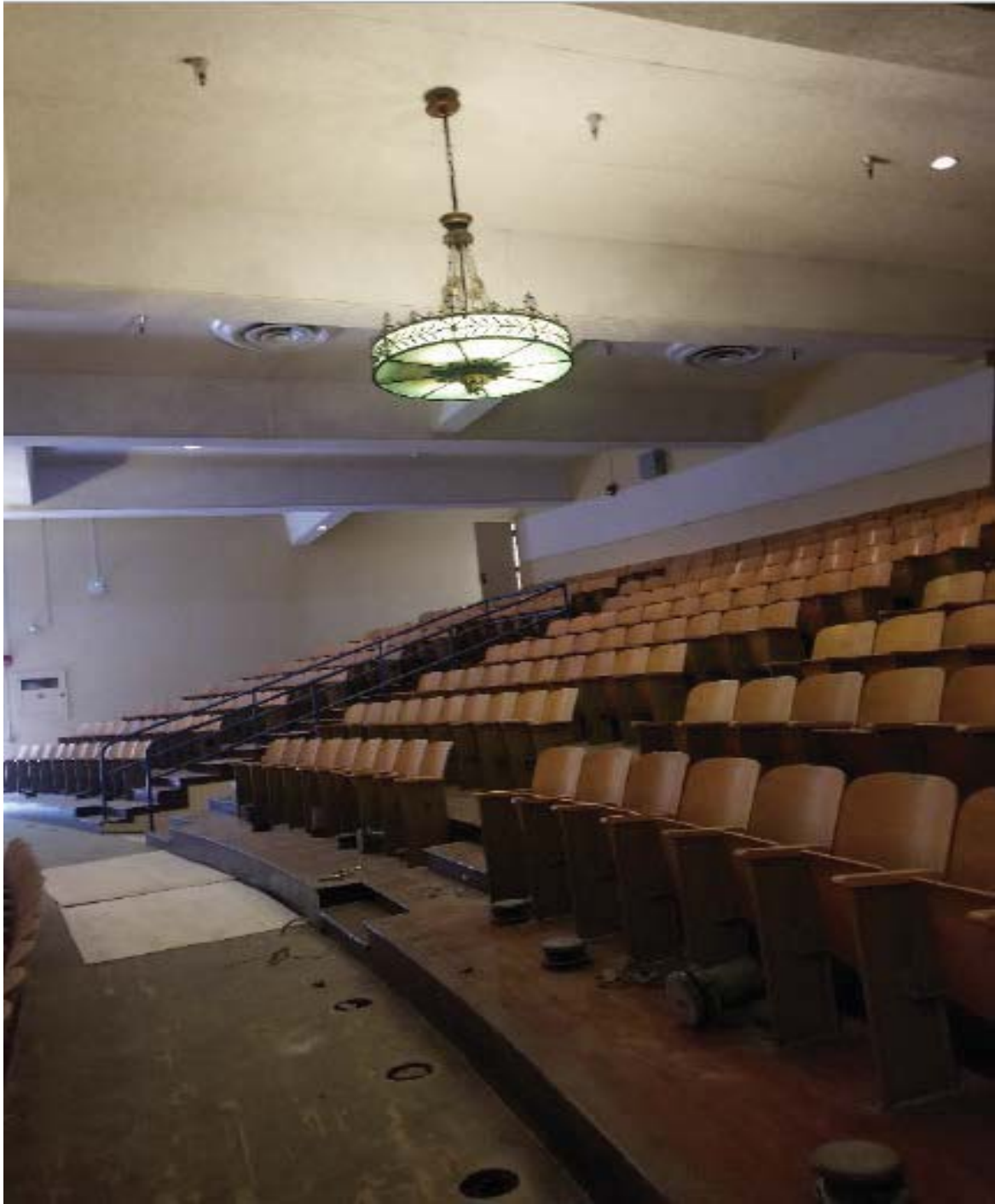
Renovation of the Auditorium – 2 nd Level
