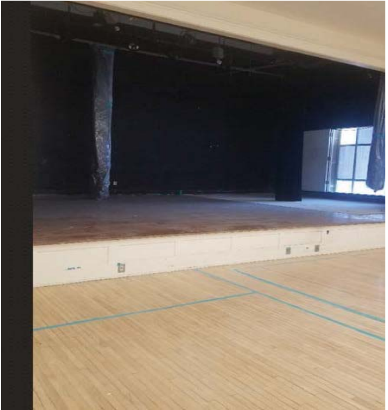
Renovation of Rehearsal Room in the Auditorium
