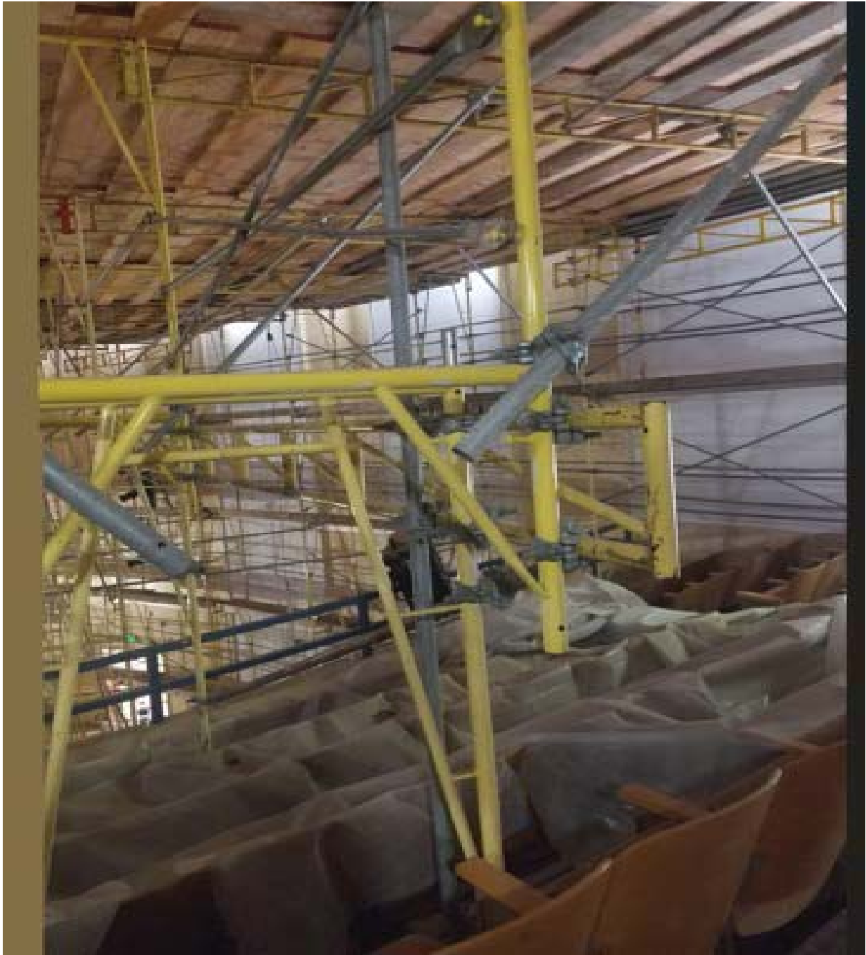
Auditorium Interior 2 nd Level Renovation in Progress
