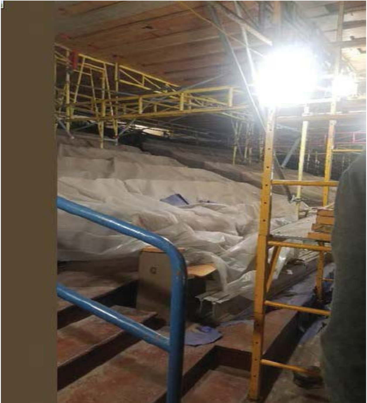
Auditorium Interior 2 nd Level Renovation
