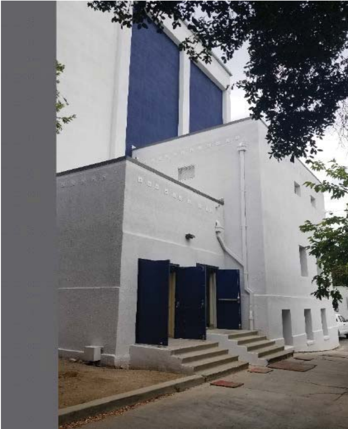
John C. Holland Auditorium – View of Completed Seismic Retrofit
