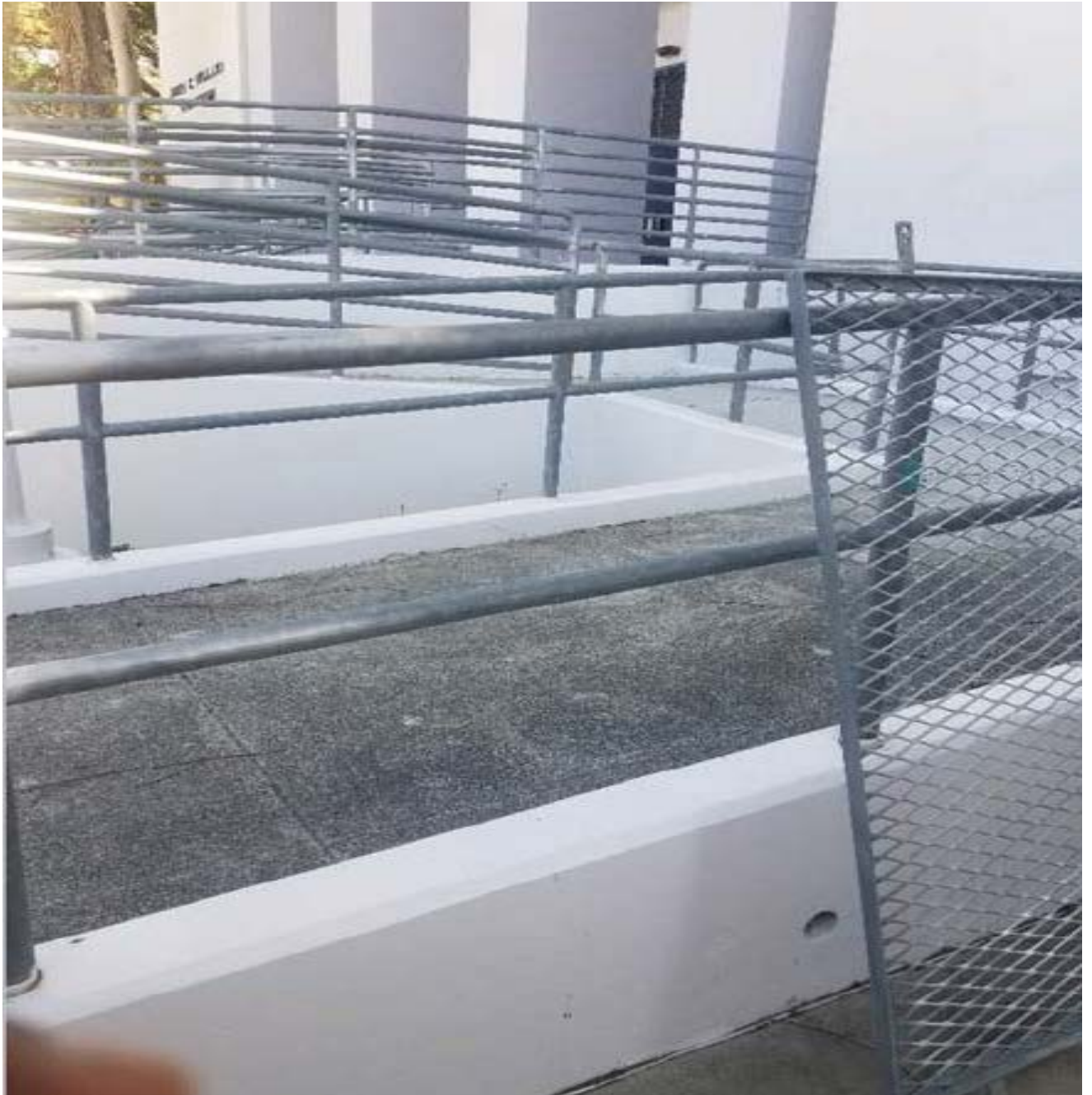
John C. Holland Auditorium ADA Walkway Upgrade
