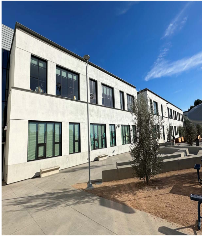
Classroom Building C - Exterior
