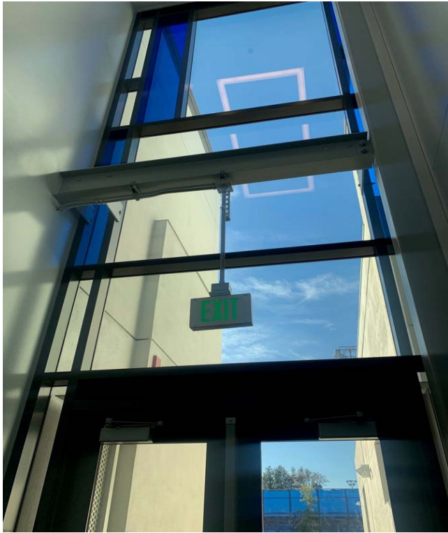
Classroom Building C – Doors & Windows
