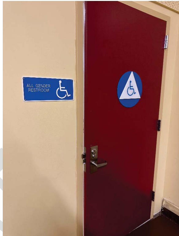
All-gender restroom door & hardware, and signage
