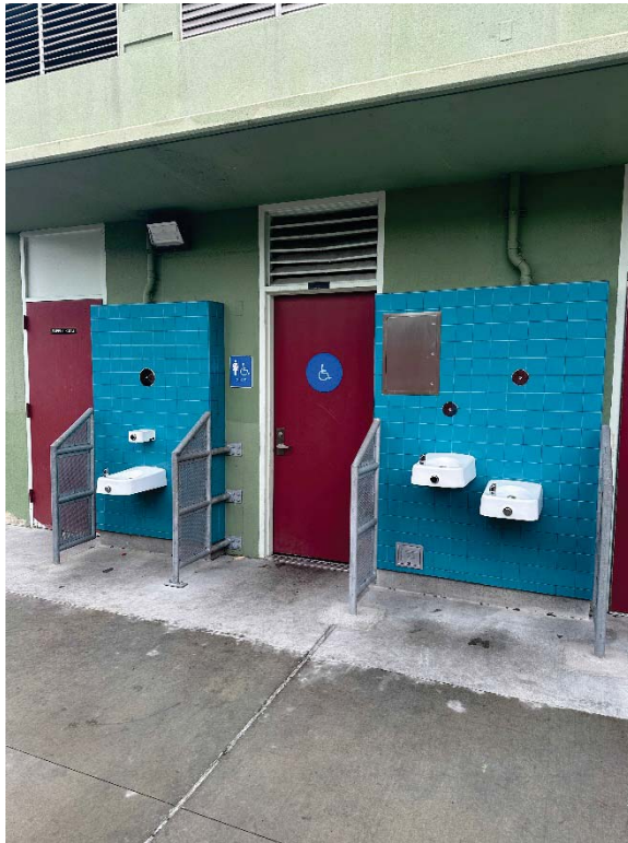
Outdoor drinking fountains and railings
