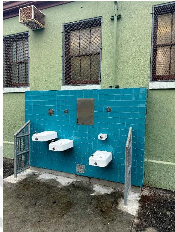
Outdoor drinking fountains and railings
